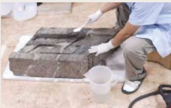
Photo 9. Washing work before reinforcement
