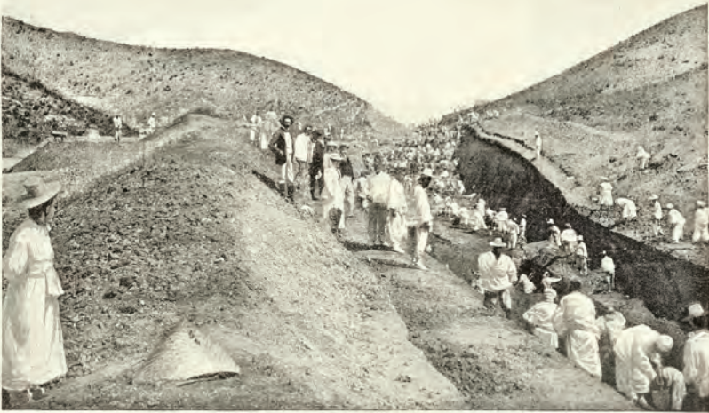
02 AMERICAN RAILWAY CONSTRUCTION IN KOREA.—DEEP ROCK CUT BETWEEN SEOUL AND CHEMULPO.
